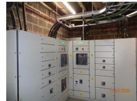
**New main LV panel** situated adjacent to the existing LV panel within Core 18 substation. (£100,000)
